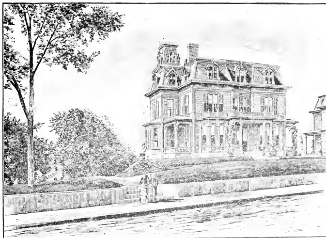
RESIDENCE OF S. C. NEWHALL, HIGHLAND SQUARE.
